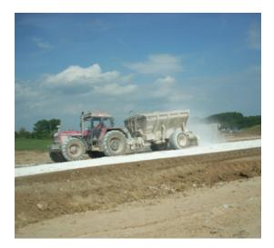
Figure 4.8 – Tractor pulled lime spreading (© Carmeuse)
