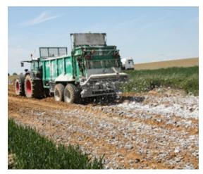
**Figure 7.16 –** Before and after treatment; lime spreading (© Nonet)
