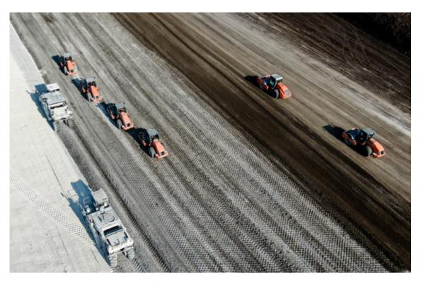
**Figure 4.23 –** Mixing and compaction operations (© Carmeuse)
