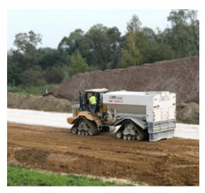
**Figure 4.9 –** Towed lime spreader (© Lhoist)
