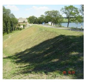
Figure 7.15 – Reconstruction of the 15 m high protection dyke at Hvezda (Czech Republic) using lime treatment of the sediments, after the floods of 2002 (© Lhoist)
