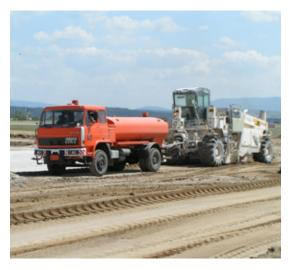
**Figure 4.20 –** Pulvimixer pushing water silo truck (© Carmeuse)
