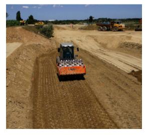
**Figure 4.22 -** Smooth drum roller / Padfoot rollers (© Lhoist)
