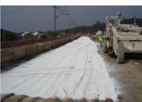
As with the Czech case study, the work was performed by half-trackbed while allowing train traffic to continue on the other line at 80 km/h. The reduced construction period, taking into account the limited space on site, was a highly valued benefit of the use of lime treatment. A rate of 200-250 m per day was achieved. Thanks to this modernisation work, it was possible to increase the train traffic speed to 170 km/h and even 220 km/h on some sections.
