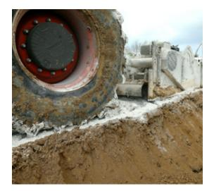
The mixing strips are about **2 or 3 m** in width. The binder must be fully mixed with the soil at all levels of the layer to be treated. Mixing can be performed to a depth of **50 cm** by large-scale mixers and **25 to 30 cm** by smaller units.
