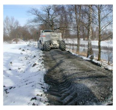
**Figure 7.9** – Lime treatment in cold conditions (© Lhoist)
