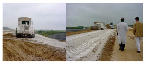
**Figure 7.2 –** Lime treatment on HSR sites (© Lhoist)
