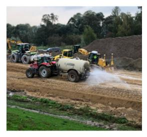
Figure 4.7 – Water addition to the surface before lime addition ( $\mathbb{Q}$  Lhoist)
