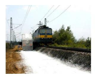
**Figure 7.5 –** Lime treatment on railway structures (Puiatti, D. & Robinet, A., Georail 2011)
