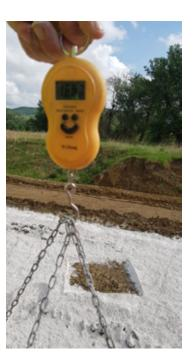
Figure A1.20 - Weighting lime on site (© Carmeuse)
