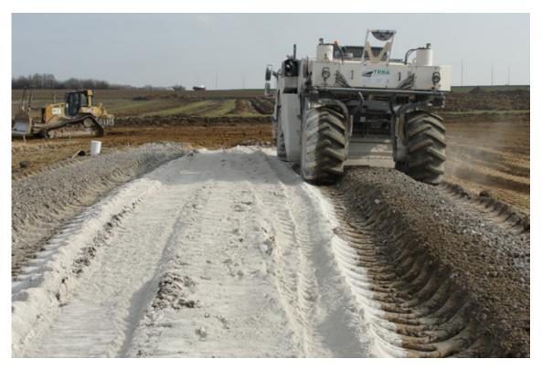
Figure 4.21 - Pulvimixer in action on clay (© Lhoist)
