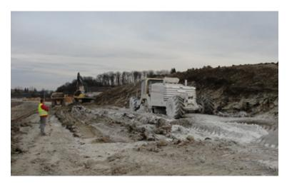
Figure 7.21 - Soil treatment operations (© Terdouest)
